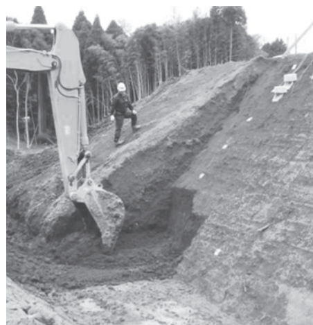
Photo 3 Overview of vertical cutting in prototype model test. バックホウを用いた切土の様子
