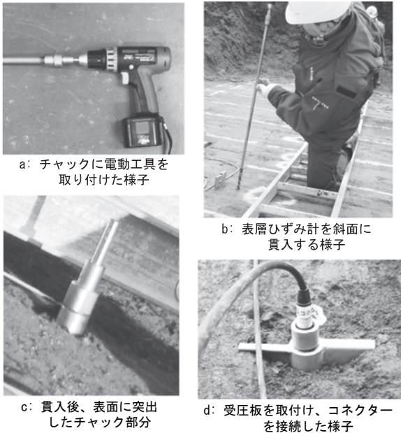
Photo 2 Process at installation of SPS. 表層ひずみ計 (SPS) の設置状況
