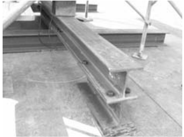
Photo 1 Fixing of H-shaped steel and 20 m 3 vessel. 20 m 3 容器のH形鋼との固定
