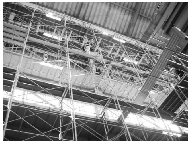
Photo.1 An experiment on the scaffold 仮設足場上での実験
