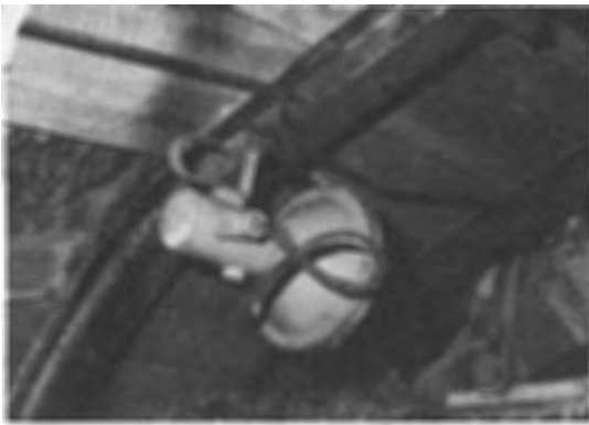
Fig.6.6 Explosion-protected incandescent lamp (Increased safety type) in using 使用中の安全増防爆形白熱電燈
