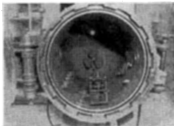
Fig. 7 A spark producer installed in an oxygen-compressed chamber.
