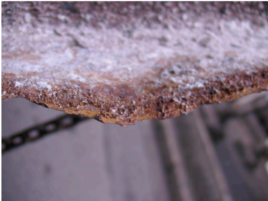
Figure 8: Ruptured part showing apparent thinning
