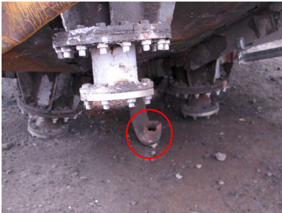
Figure 7: The 044 tank top board (blown off and separated from the tank, the original position was upside down)
