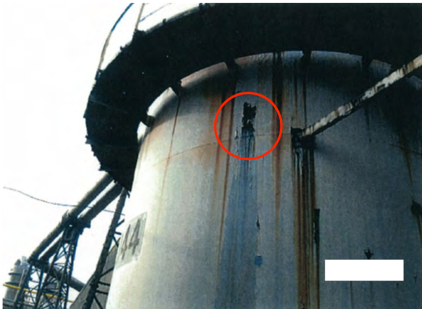
Figure 6: Oozing observed before the accident
