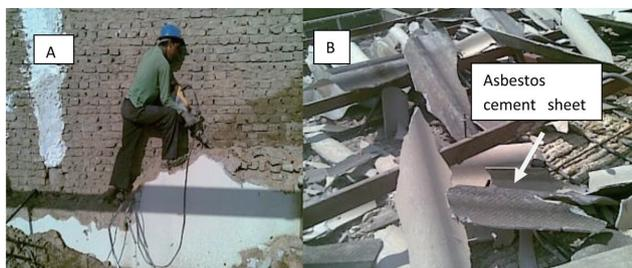
**Fig. 1.** Demolition in progress. (A) during demolition; (B) after demolition and before debris removal.
