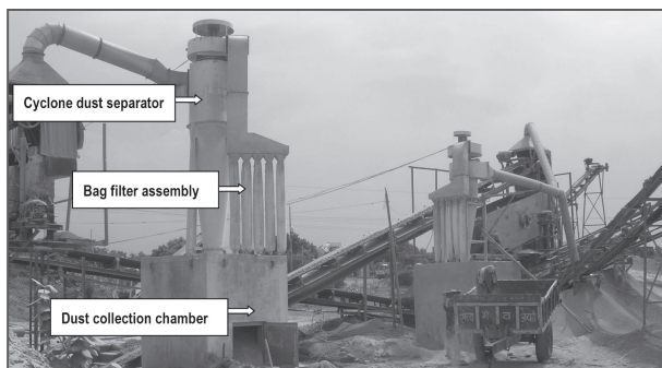
Fig. 2. The dust control system.
