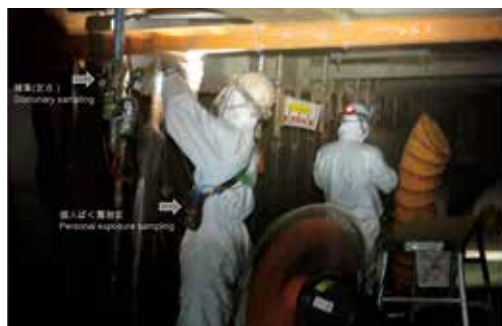
化学物質ばく露による労働災害の原因調査 (道路橋延命工事の鉛入り防錆塗料剥離作業における鉛濃度測定) Exposure monitoring for investigation of an occupational accident (evaluation of lead exposure during removal of lead-containing paint from a steel beam of a road bridge).
